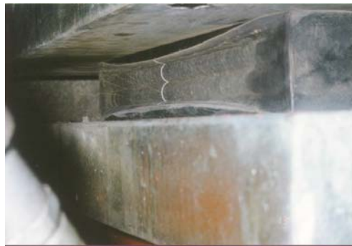
Fig. 26: Newly replaced laminated elastomeric bearing at Ahmad Shah Bridge
